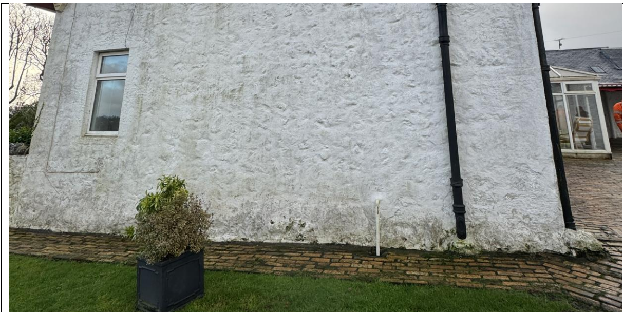
Figure 27 image of side elevation showing what appears to be rock forming the exposed foundation
