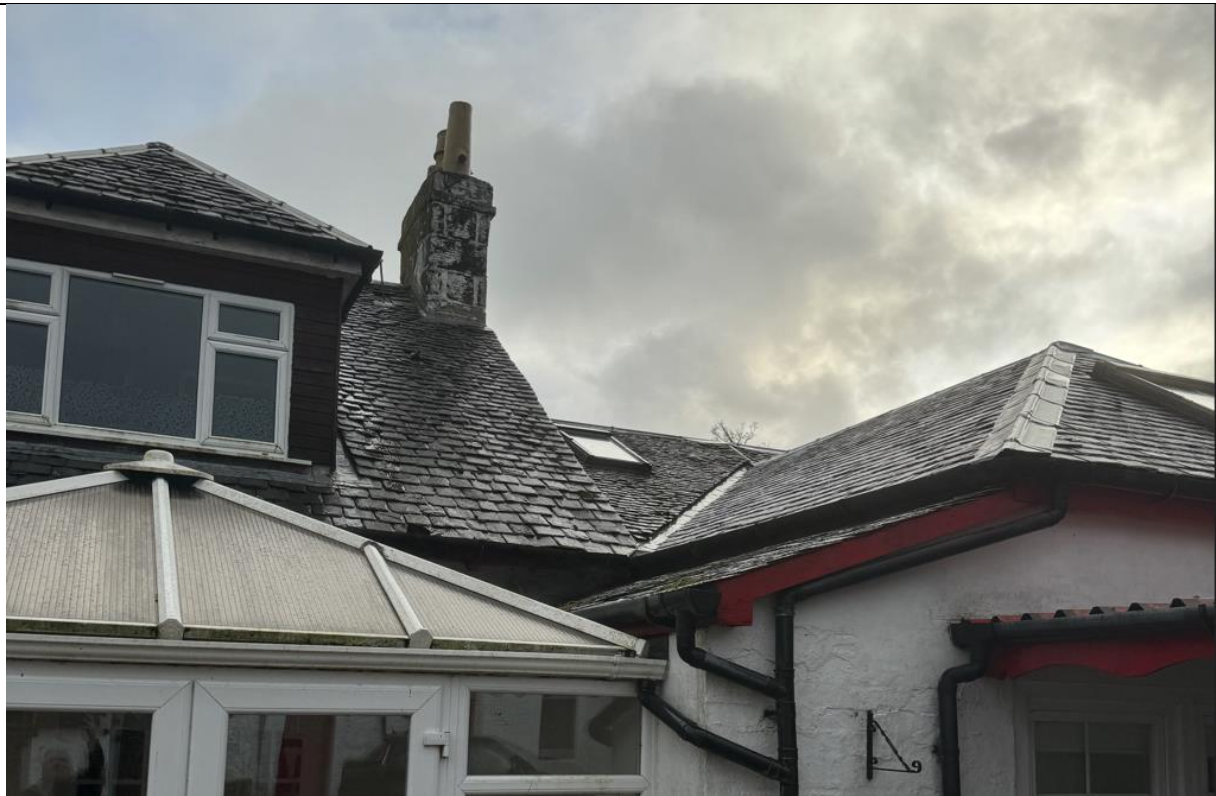
Figure 7 Images of external roof link between house and stables showing slate covering and metalworks
