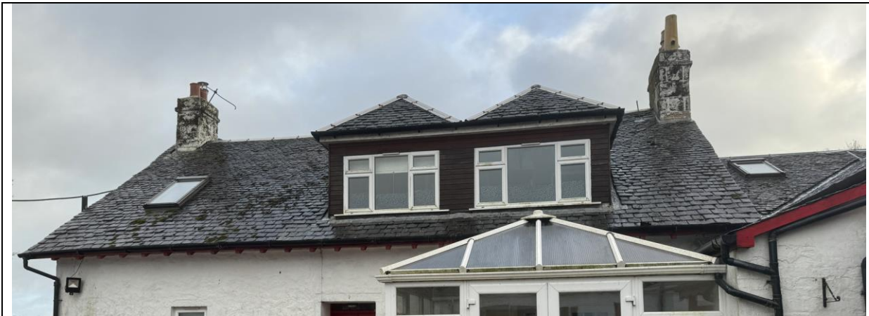
Figure 5 Images of external roof showing slate covering, dormers, chimneys and metalworks
